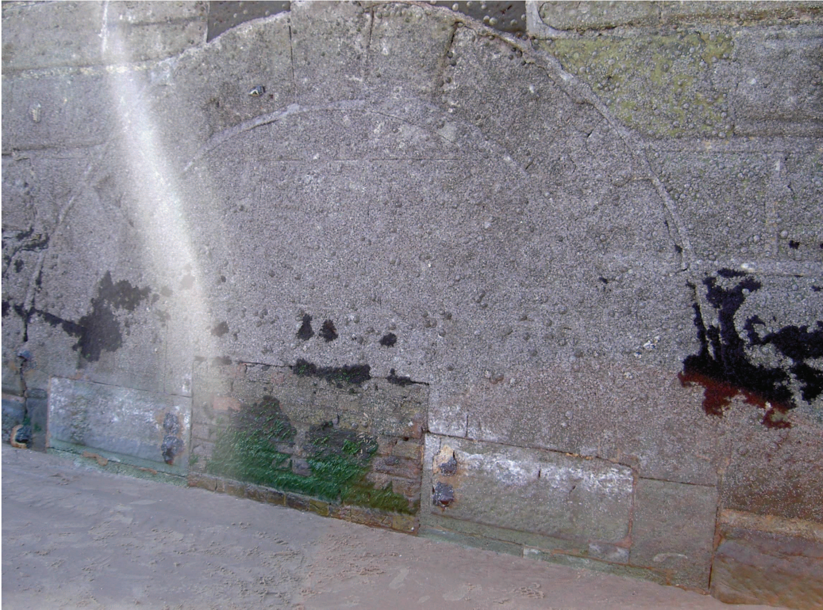
Margate Harbour Sluice –Portland Stone and Brick sealing wall to culvert viewed from outer face of Stone Pier
