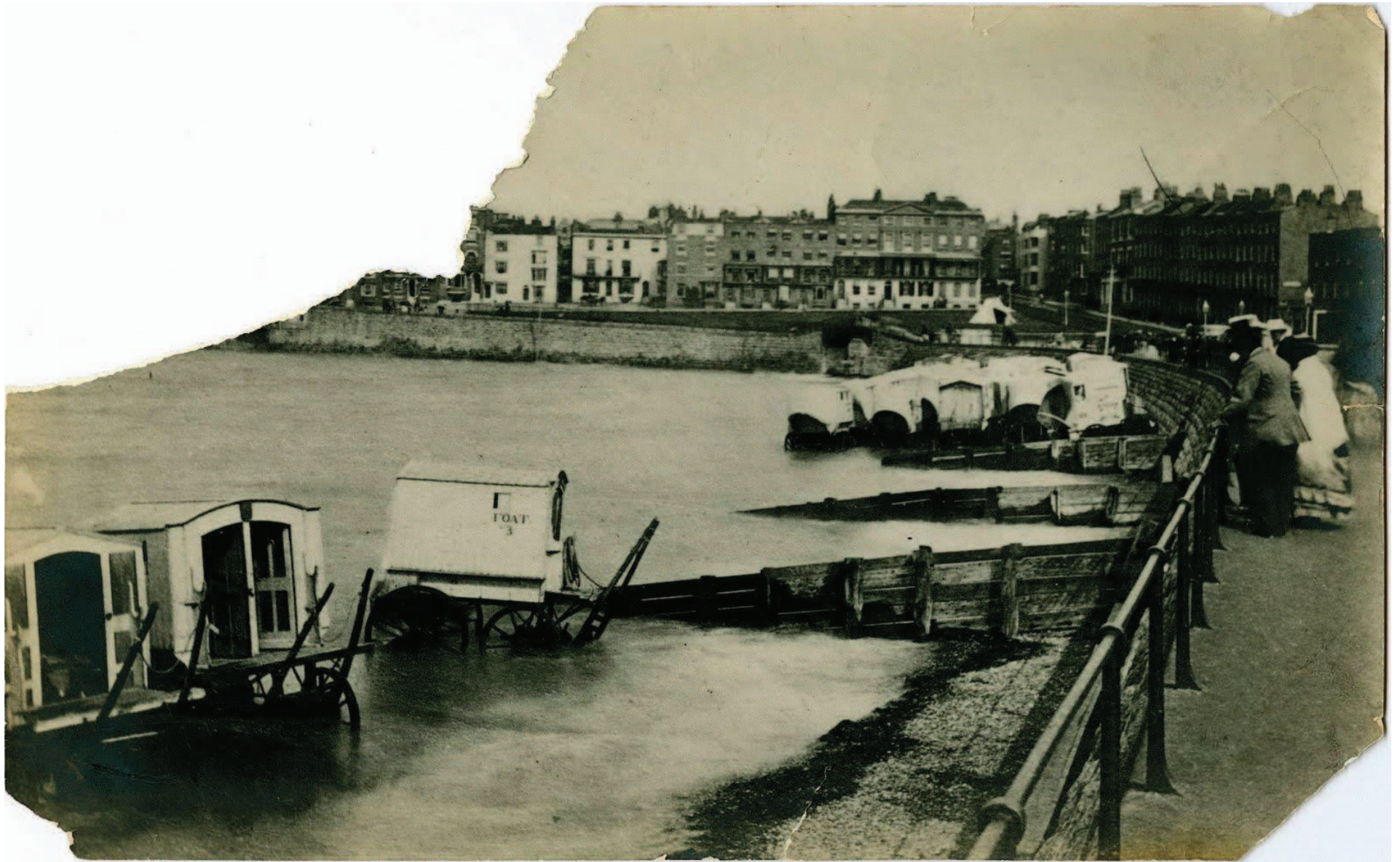
Marine Terrace before 1887 – The tide reached the sea wall twice daily under normal conditions
